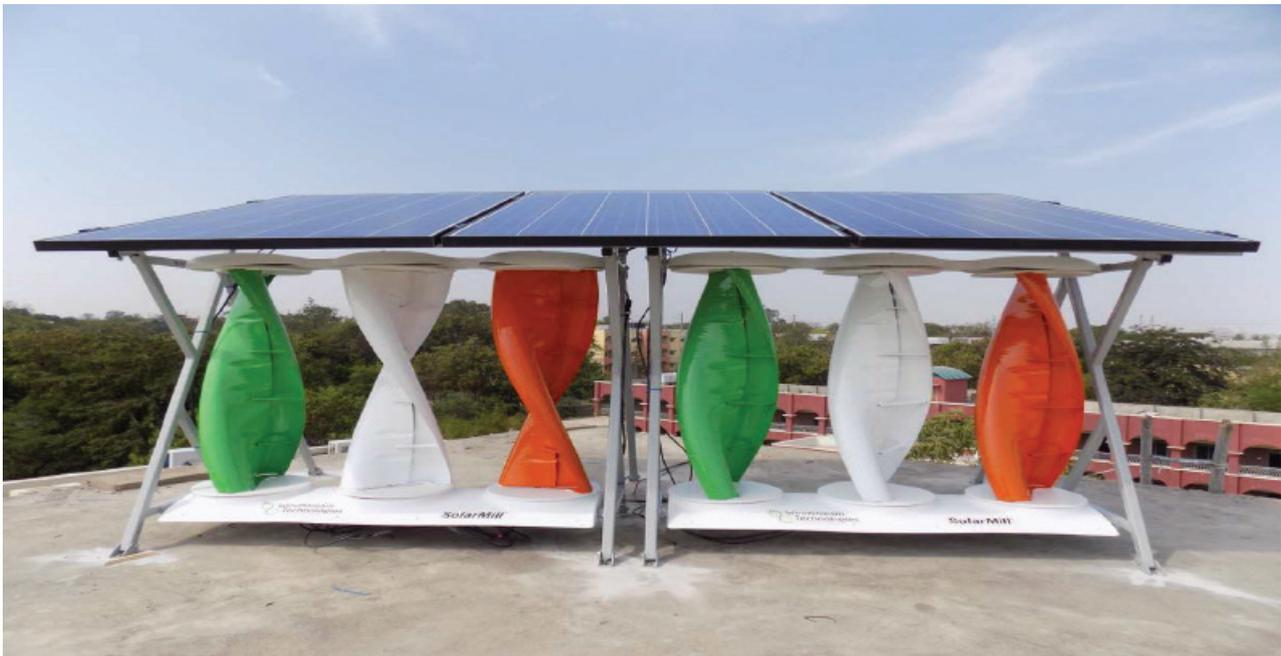
Figure 83: Solar-wind hybrid system
