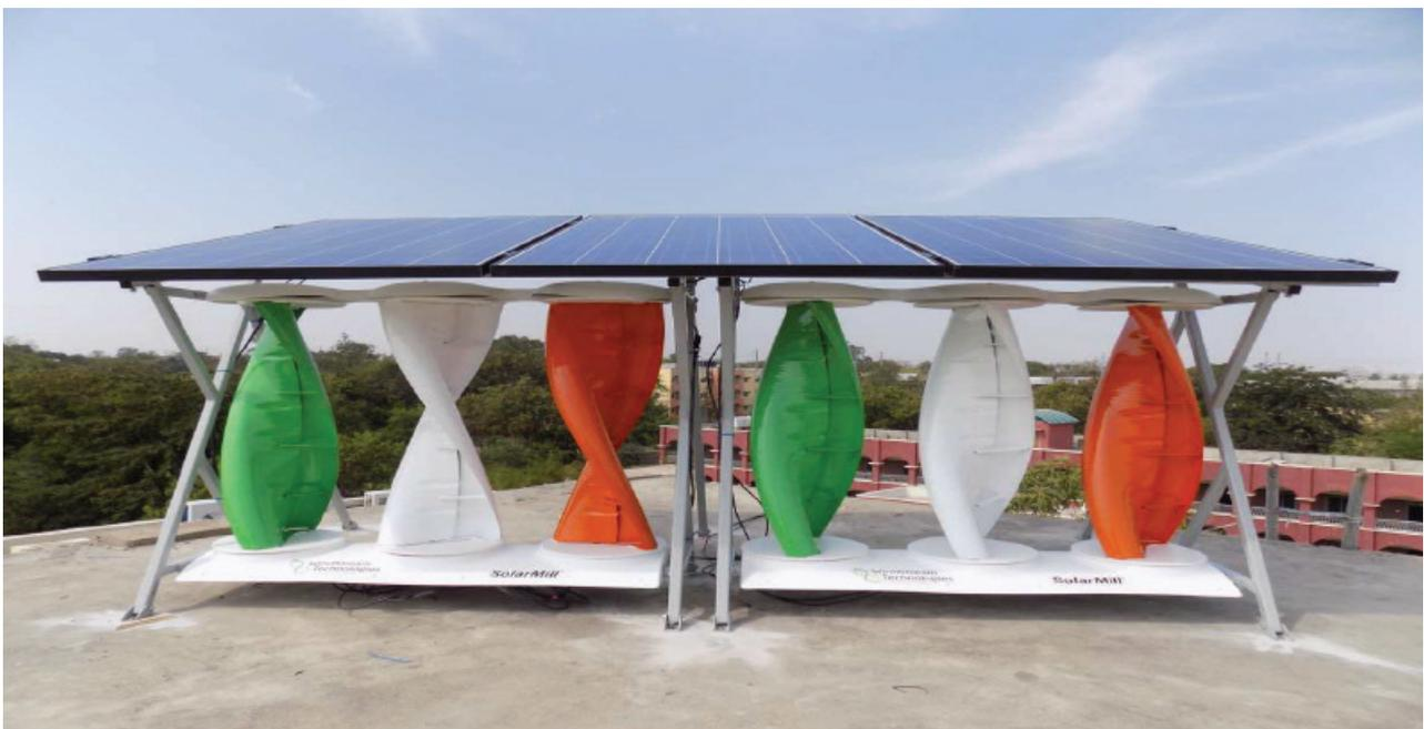
Figure 52: Solar wind hybrid system
