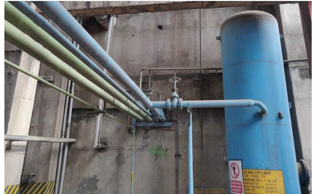
Figure 41: Existing compressed air piping
